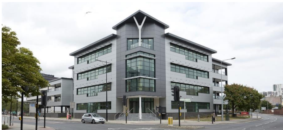
Figure 12 – Berkeley Business Centre, Connexions 159, Princes Street, Ipswich
