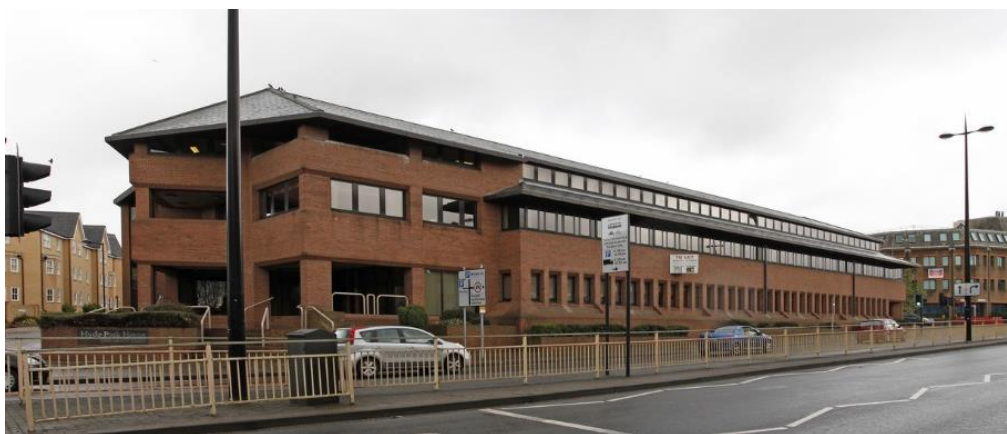
Figure 10 – Hyde Park House, 1 Crown Street, Ipswich
